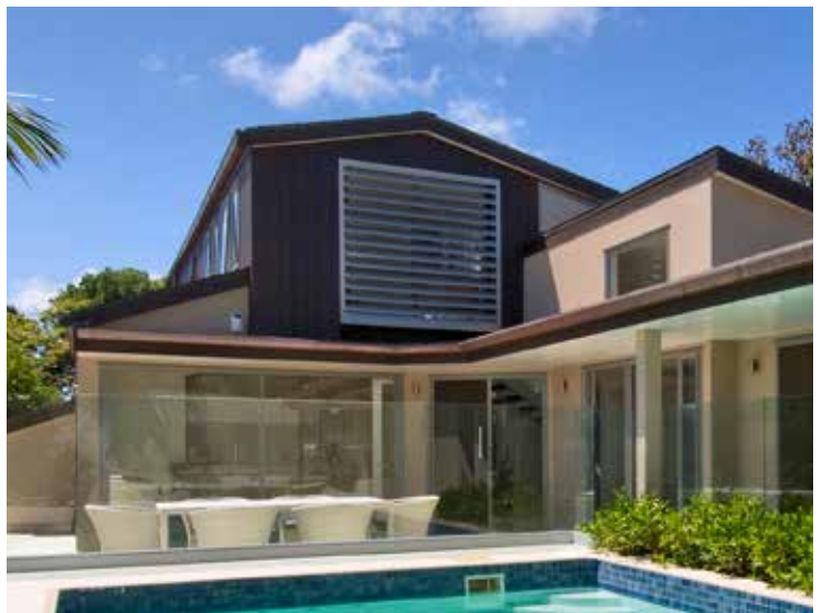
MOTORISED, VERTICAL SUN LOUVRES INCLUDING STRUCTURAL FRAME
